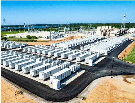
DeCordova Energy Storage Facility 260 MW/260 MWh Battery + CT Hybrid
